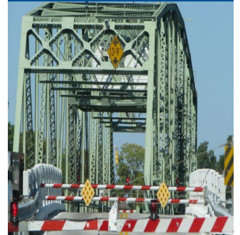
Gwynn's Island Bridge
