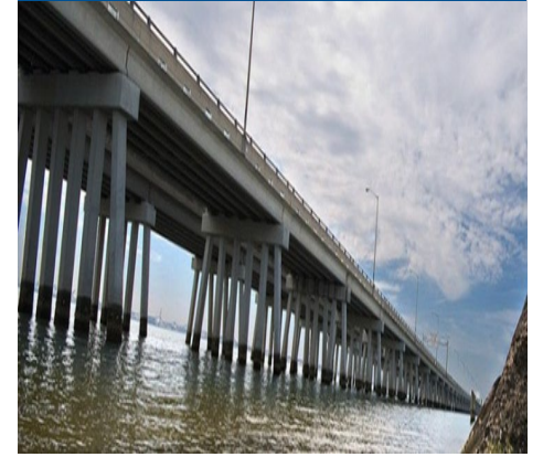
Hampton Road Bridge-Tunnel (Willoughby Bay)
